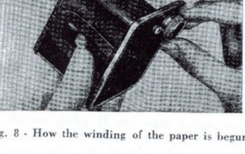
Fig. 8 - How the winding of the paper is begun
